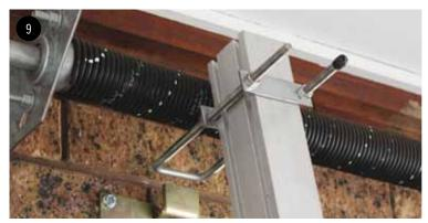
Lift and align the B&D High Wind brace, by position the U Bolt onto the bolted wall mounted top bracket.
