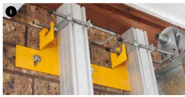
Unhook the U Bolt at the top of the high wind brace from the top wall storage mount (pull away from the wall and lift).
