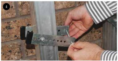
Locate and remove the wing nuts and bolts from each brace, keep handy. Swing all flat arms to a down position.
