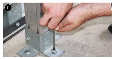
Once the brace and holes are aligned begin the process of screwing down the Floor Flange with the Anchor Screws. Ensure you screw in each of the Anchor Screws previously removed; there are three screws per B&D High Wind brace.
