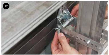
Swing all the flat arms on the brace up, so that the long end is aligned with the metal hinge. The previously removed wing nuts and bolts can be fitted through the arms and the hinge. Once the nuts and bolts are tight ensure the brace is secure. For the remaining B&D High Wind braces repeat the process.
