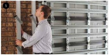
Pick up the B&D High Wind braces stored next to the door. Ensure you have a firm grip on the brace and remember to lift with a straight back whilst bending at the knees (caution braces weigh 15kg each).
