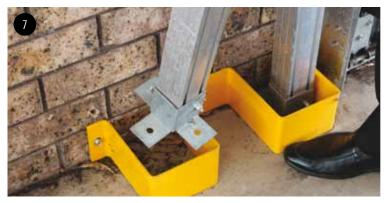
Remove the brace from the footing case (by lifting vertically).
