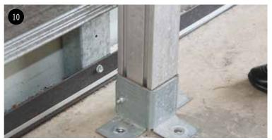
After the top bracket and the U Bolt are connected, align the Floor Flange with the anchor holes in the floor.
