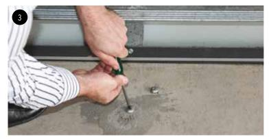
Firstly, remove the floor anchor screws, by unscrewing them anti clockwise. There are three screws per B&D High Wind brace.
