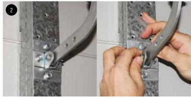
Disengage the Hockey Stick and pin, by unclipping the R clip and sliding out the stick. (This may not be necessary on doors with no centre brace). Be careful as the Hockey stick may swing backwards.
