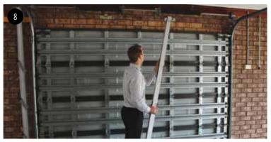
Once the braces have been removed from the wall storage mount, move them into the door bracing position.
